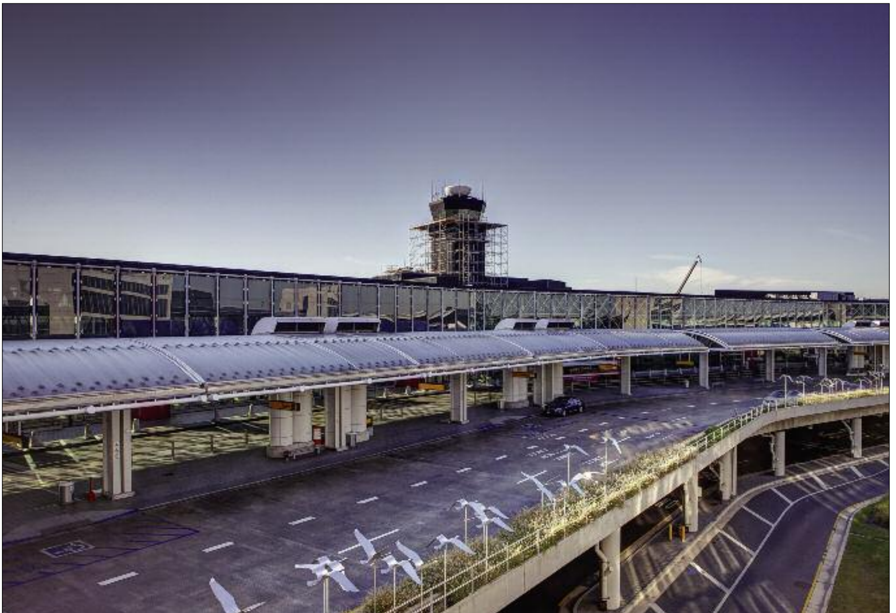
BWI Tower Glass Replacement — Photo: Kevin Weber
